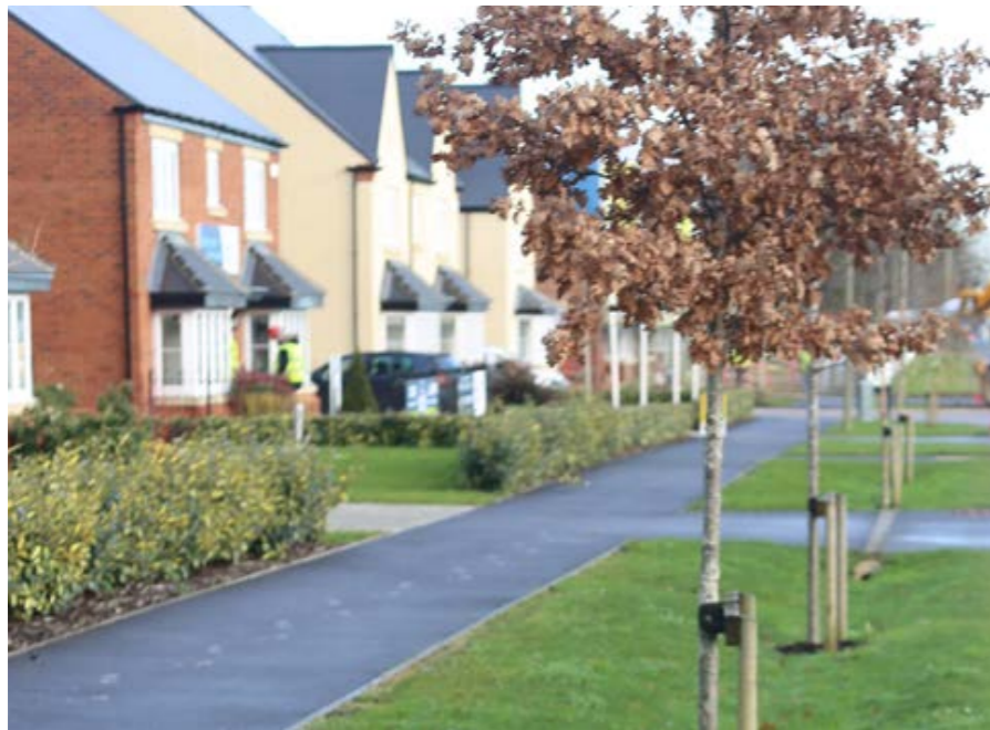
Swale & Shared Footway- Heyford Park, Oxfordshire
